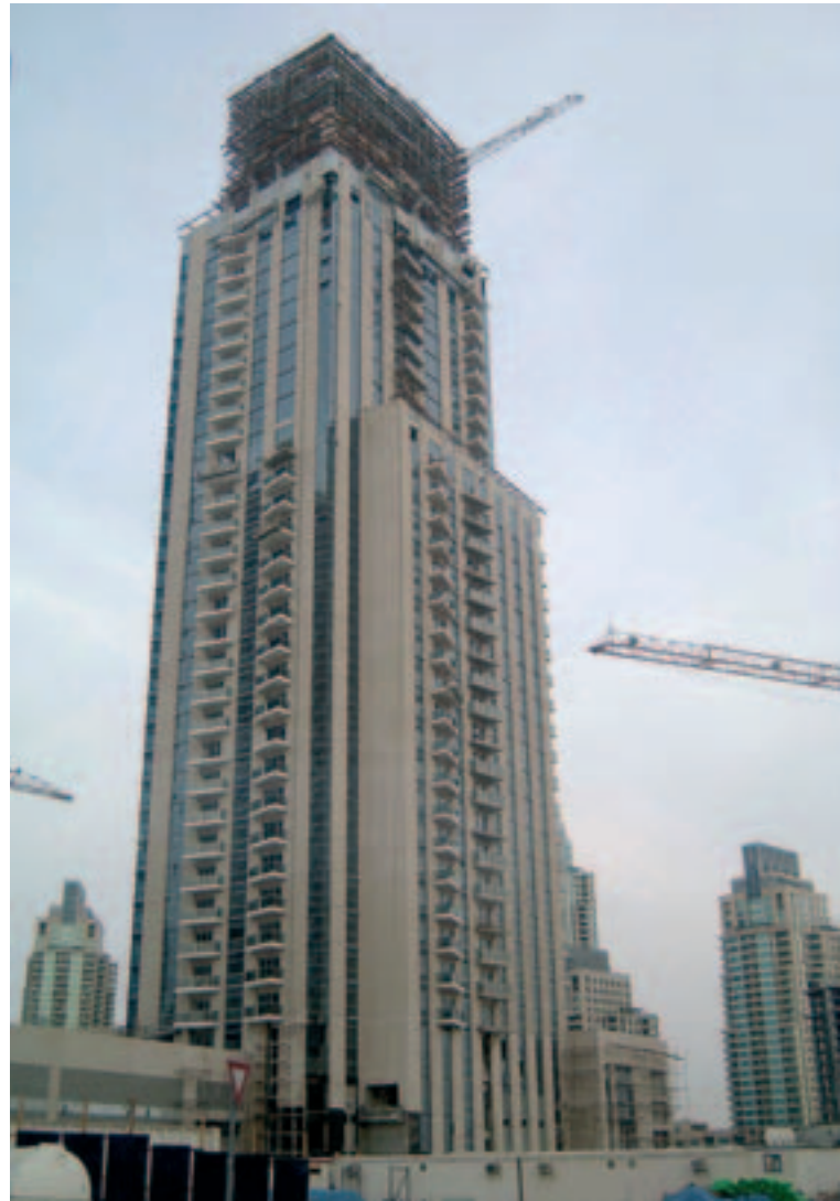
This residential building in Dubai Marina is covered by around 20,000 sq meters of wall panels. The surface is in white concrete with exposed white stones.
