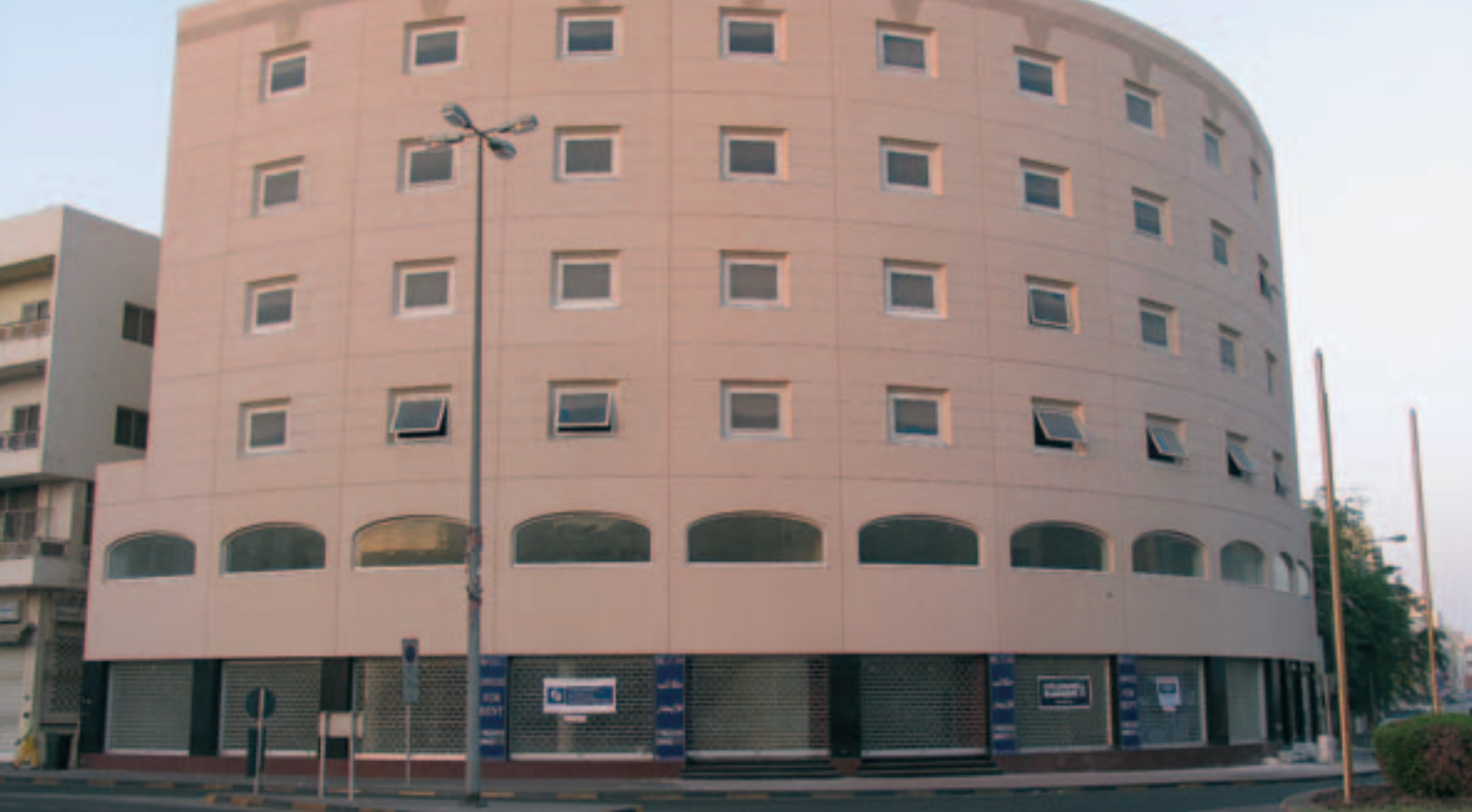
The round shape of this commercial building in Bahrain is formed by 56 advanced wall panels, each following the curve of the building.
