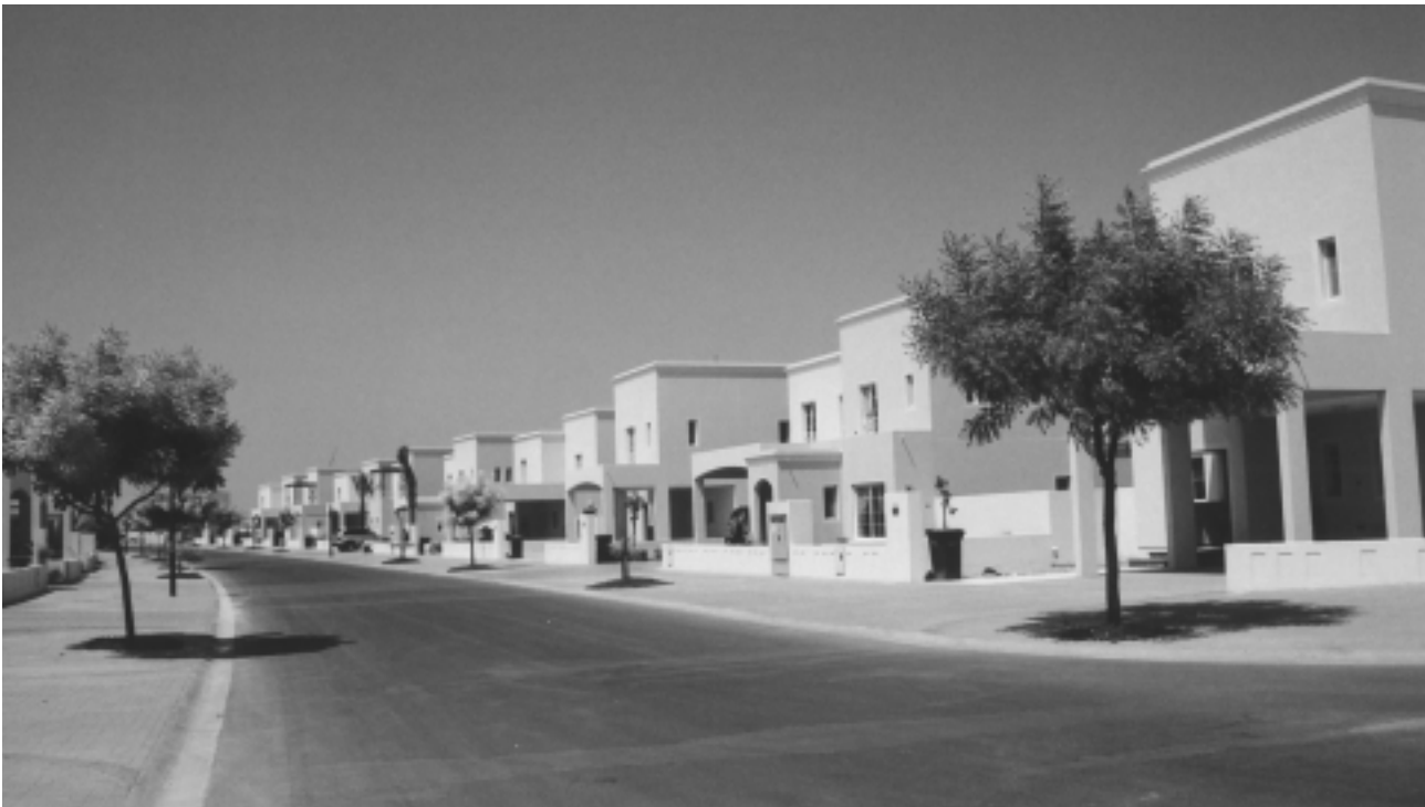
For The Meadows housing area in Dubai, United Precast Concrete, Dubai and Abu Dhabi, has supplied and erected façade panels, hollowcore slabs and stairs for 421 villas.
