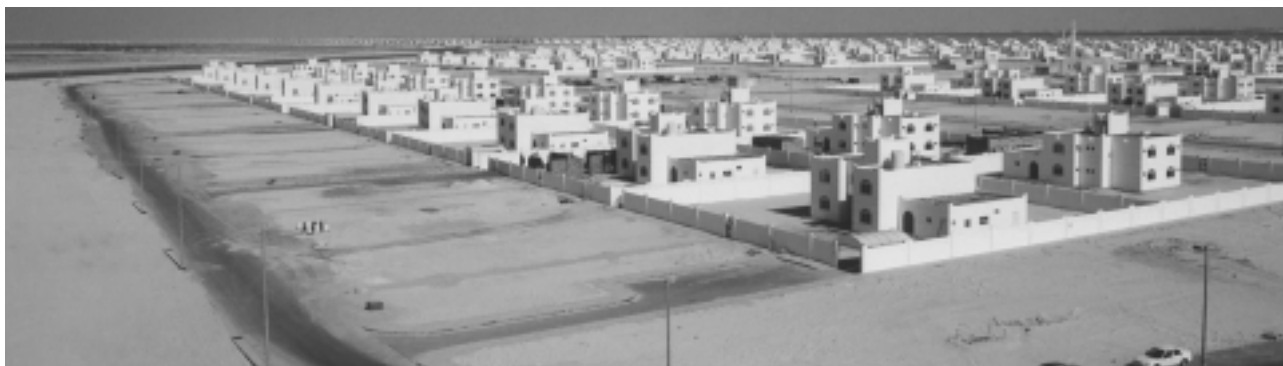
Part of the desert has been allocated for the building of 230 villas in Abu Dhabi. All supplied by the local BPC Group plant.
