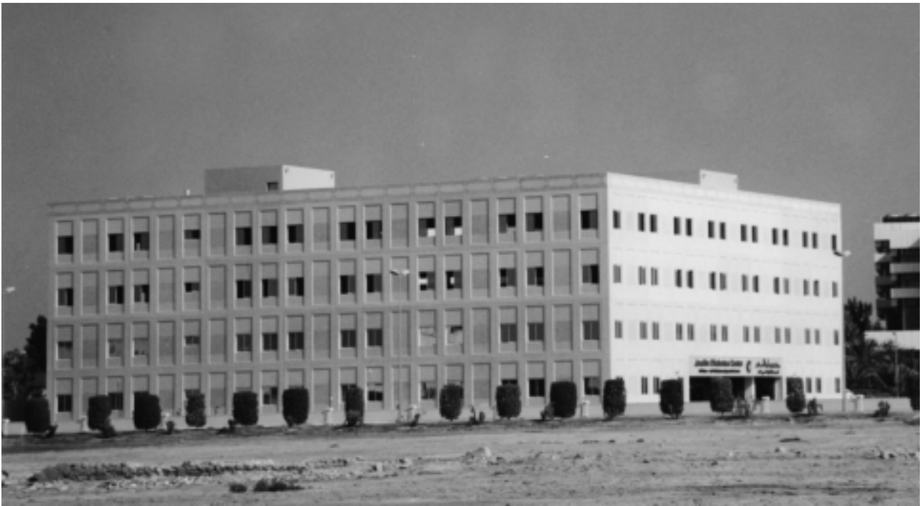
For Joslin Diabetes Center in Bahrain, 200 mm hollowcore slabs and white, sand-blasted and insulated façade panels have been supplied.
