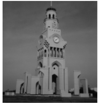
Riffa Clock Tower offers fine evidence of the sophisticated production technique applied by Bahrain Precast Concrete.
